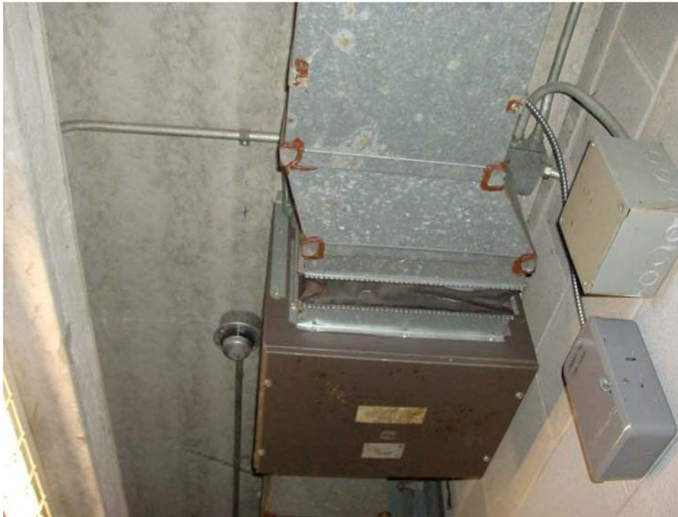
Photograph 2: View of flexible duct joint material that could not be sampled without damaging the seals on the unit.
